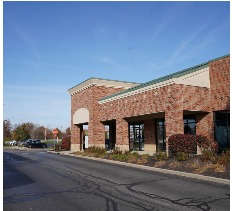
View Facing North
