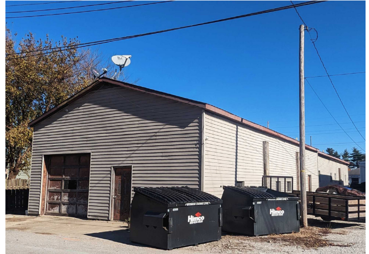
Back alley view of warehouse
