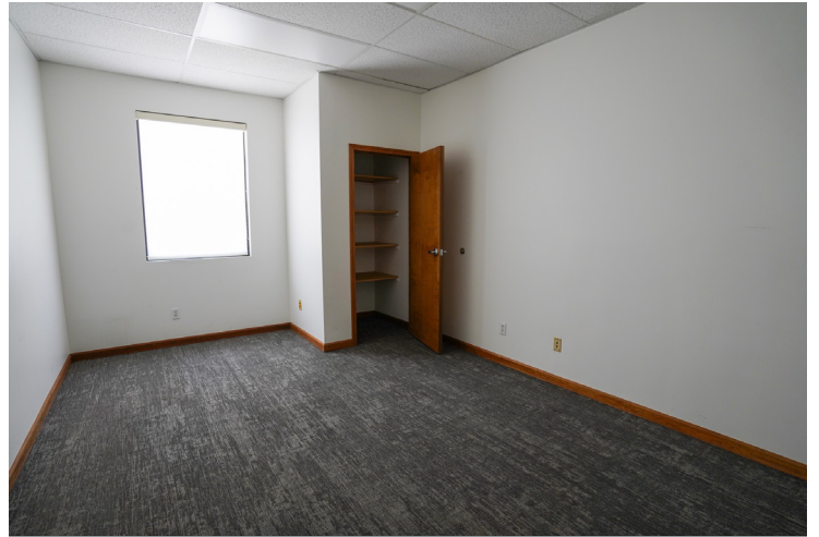
2nd-floor office space
